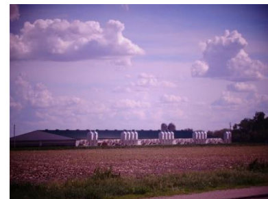
Example of an Animal Confinement Building
